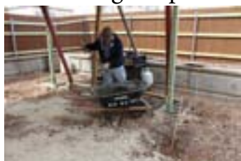
Mixing the concrete to secure the awning
