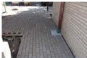
Installing the patio
